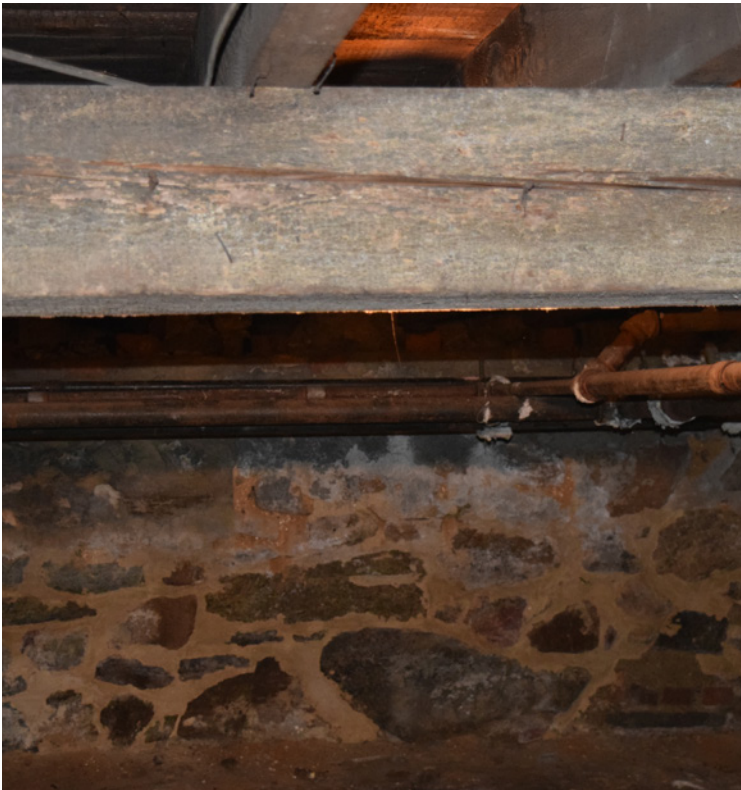
Unventilated Crawl Space with checked beam
