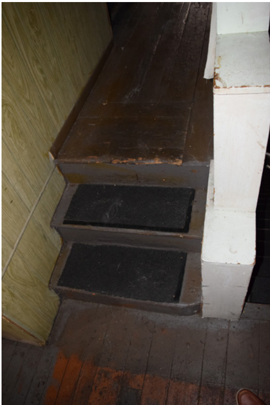
Unsafe split level stair
